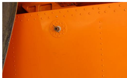
Level indicator Tank No. 3.
